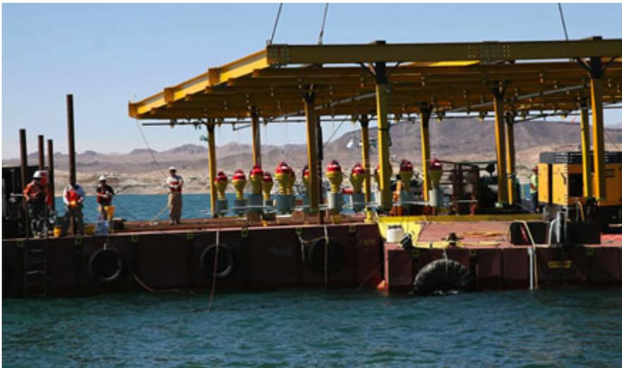
*Shows explosive frame ready to be lowered and accurately positioned using sonar on board the Falcon.*
